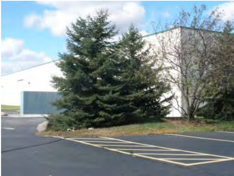
Southeast corner of building; camera looking northwest (Loading dock area and dumpster screen)
