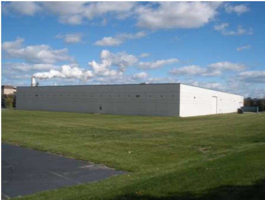
Southwest corner of building; camera looking northeast (View from meat packing plant)
