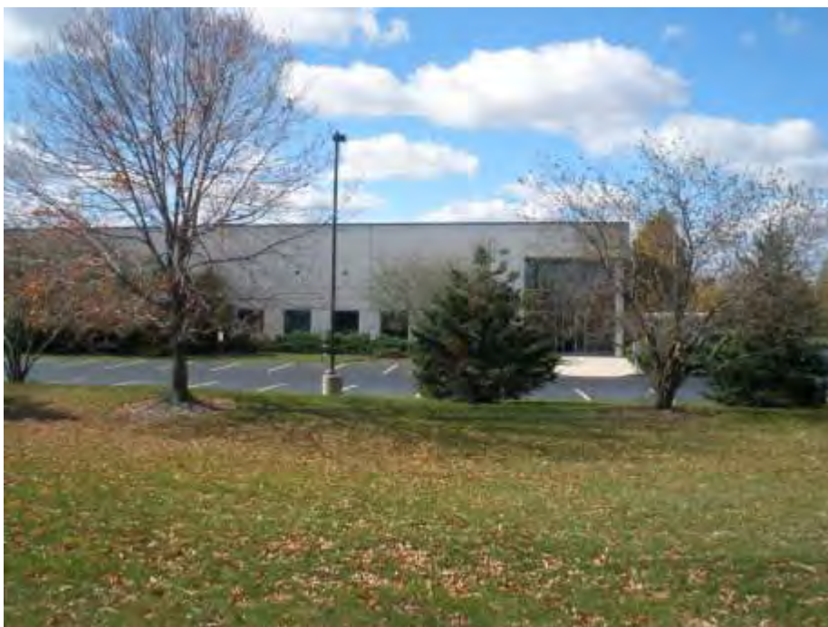
East face building entry looking West (View of Building from 88 th Avenue)
