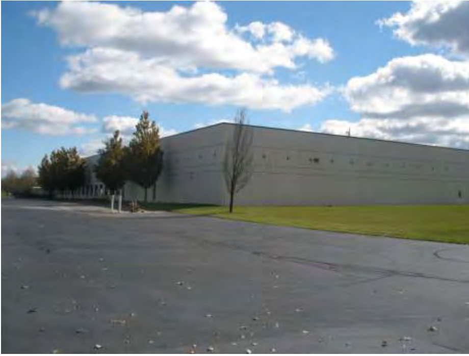
Northwest corner of building; camera looking southeast
